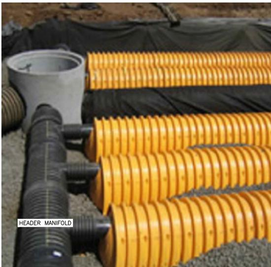
STORMTECH SUBSURFACE CHAMBERS ARE AN EXAMPLE OF UNDERGROUND STORAGE<sup>3</sup>
